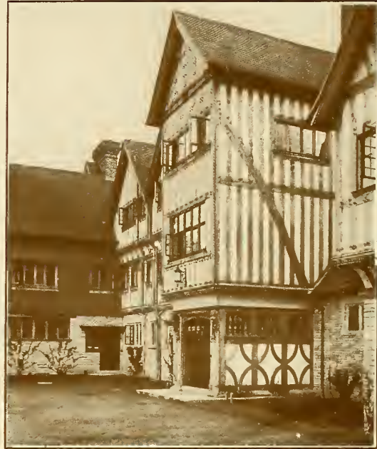
LADY BRASSEY'S HOUSE A. N. Prentice, Architect, London
